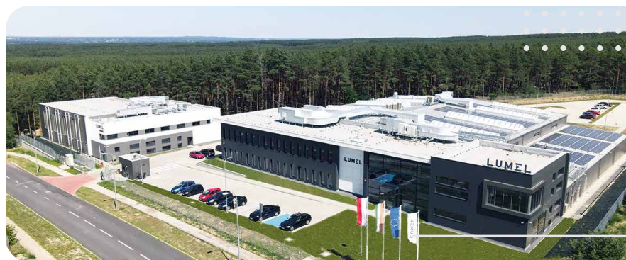
Plant area 3650 m 2 powered by Lumel solar installation.
